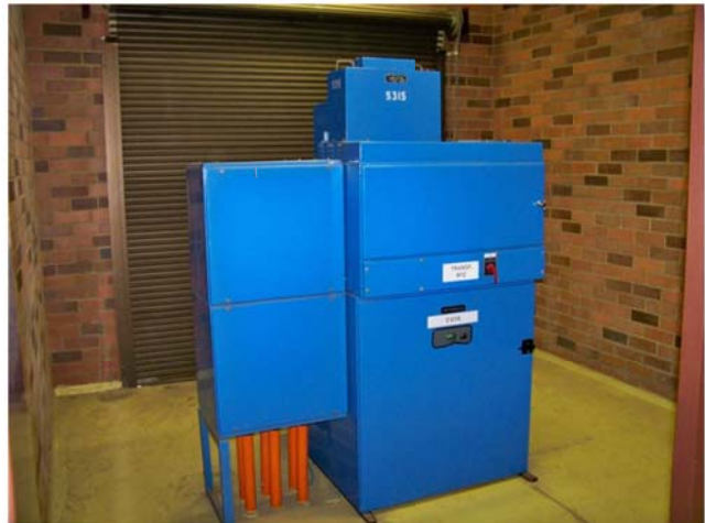
1 of 3 Reyrolle LMT 11kV transformer circuit breakers in dedicated room
