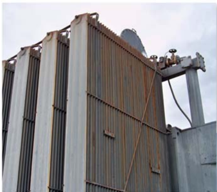
Power transformers with rusting radiator fins and oil leaks
