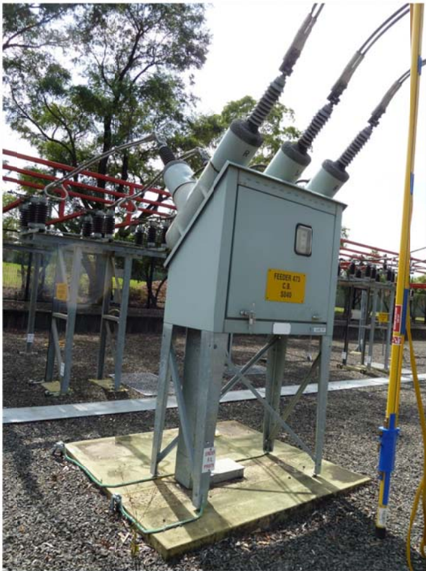
1 of 5 33kV Areva OX36 SF 6 circuit breakers to be removed to spares
