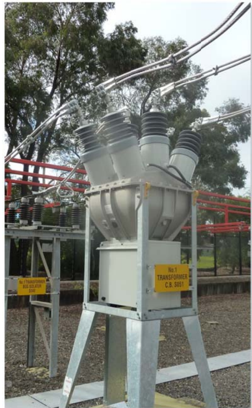
33kV Hawker Siddeley VOX SF 6 circuit breaker to be removed to spares
