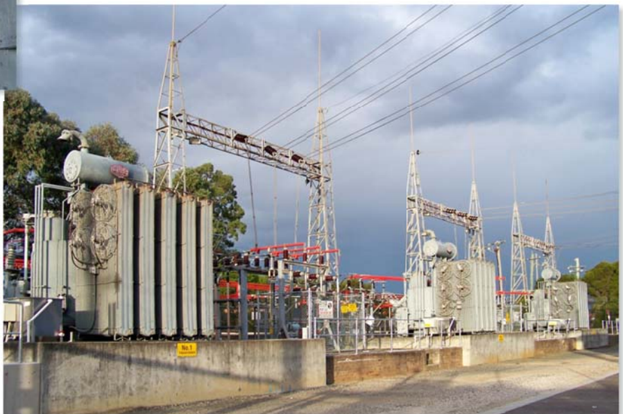
Power transformers with rusting radiator fins and oil leaks
