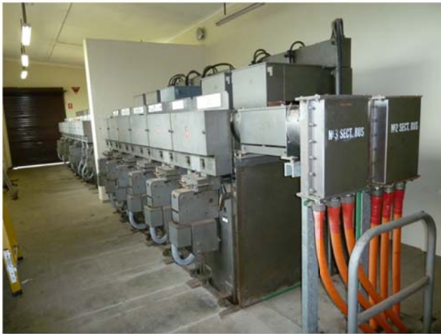
The 11kV Westinghouse HQ switchboard
