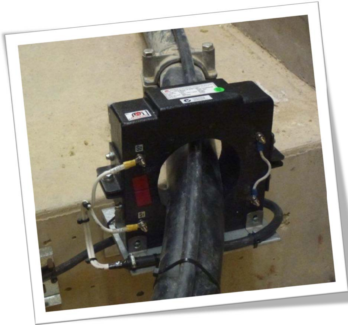
A core balance CT installed at Blackheath Zone Substation
