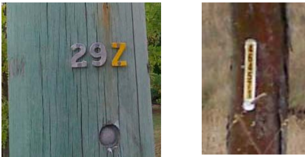
Figure 3: Pole number, disk indicator and aluminium pole number plate
