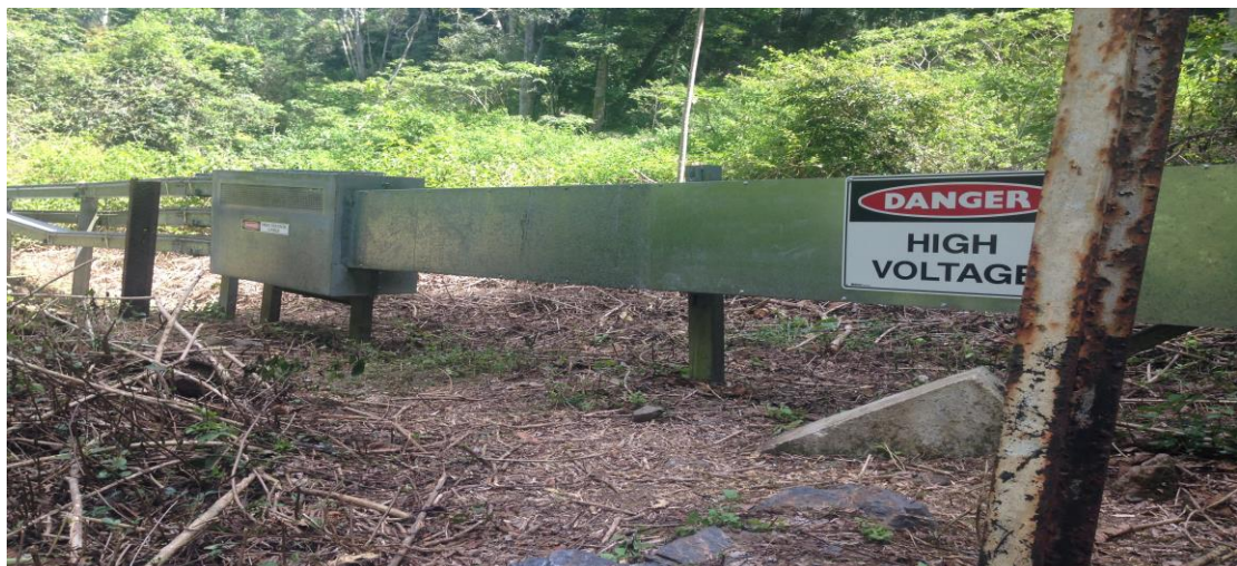
Figure 2-1: Directlink galvanised steel tray
