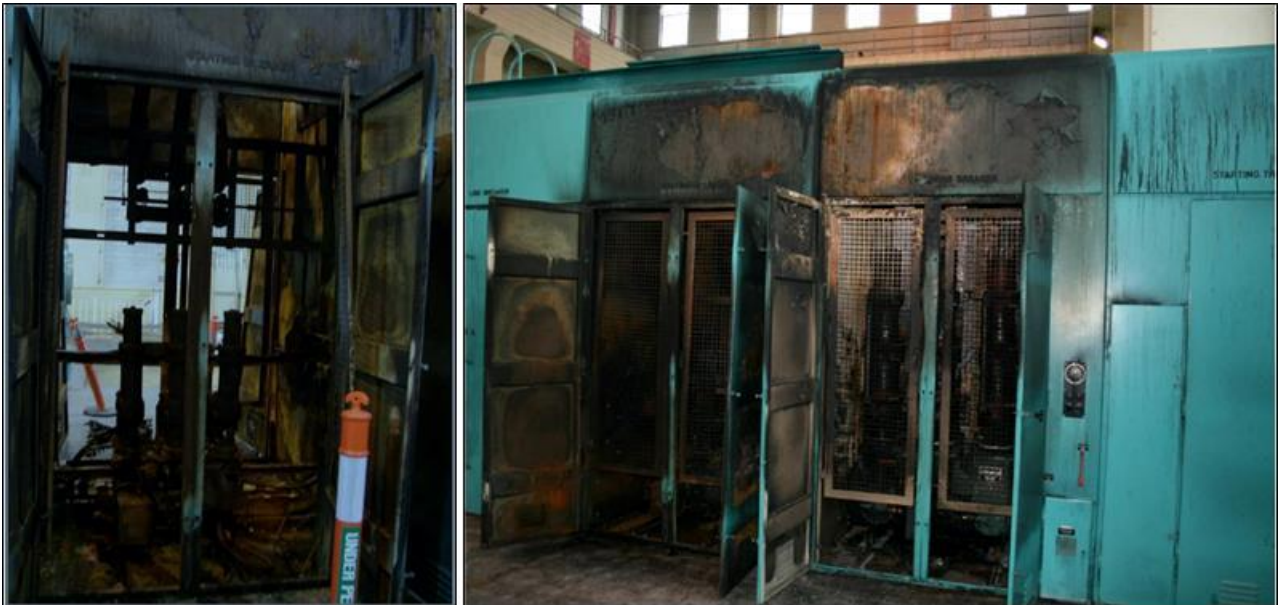
Figure 11 Example: before and after pictures of an 11kV switchboard incident (2009)
