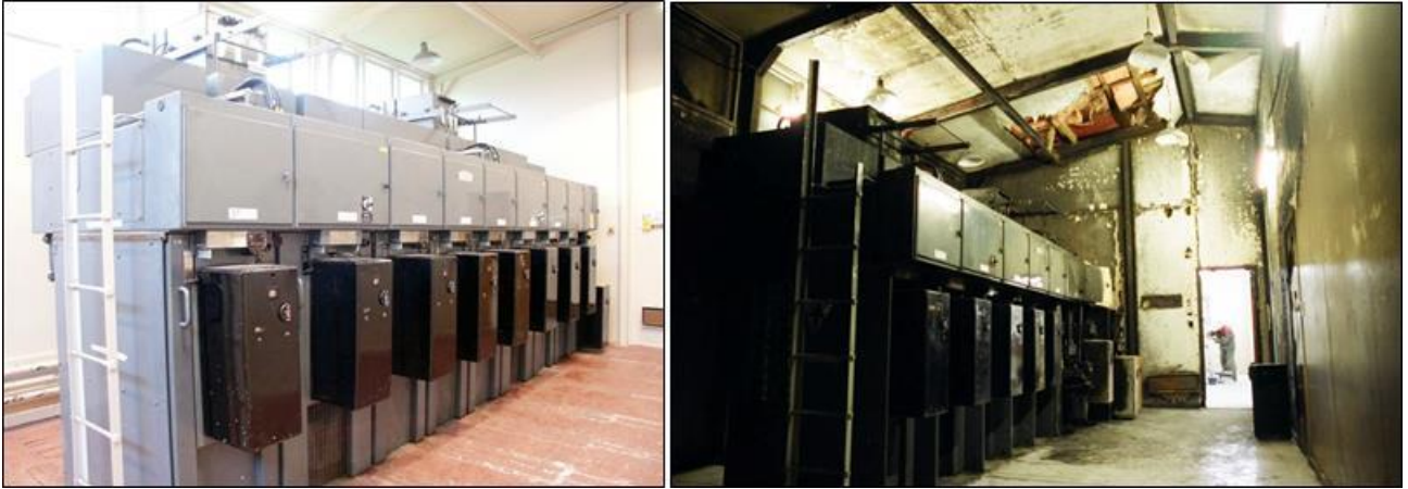
Figure 10 Example: before and after pictures of an 11kV switchboard incident (2007)
