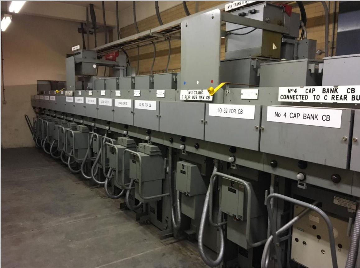
Figure 4 11kV switchgear installed at LQ zone substation
