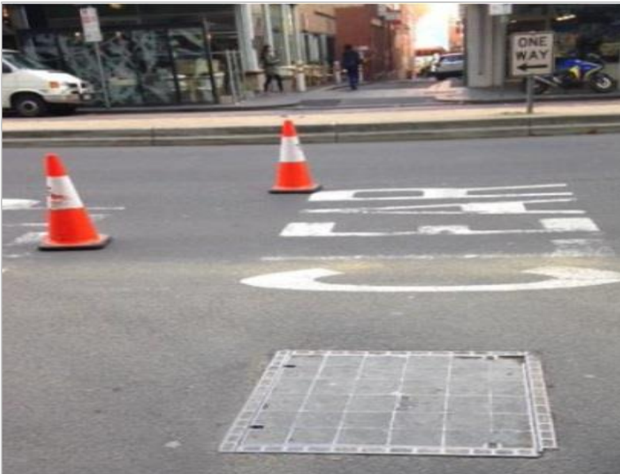
Figure 1 Example of roadway pit with Gatic cover lid
