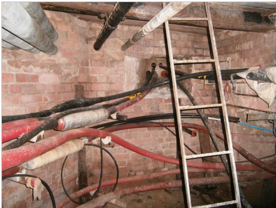
Figure 2 Typical cable pit internal arrangement
