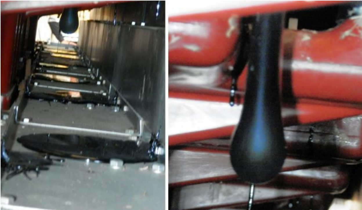
Figure 13 Example: void in compound insulation in bare busbar highlighting failed integrity of electrical insulation (2015)
