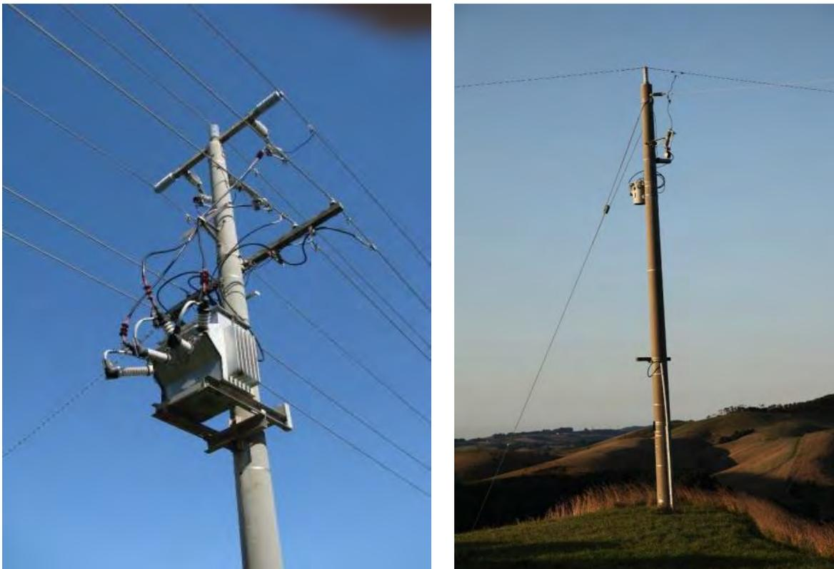
**Figure 2: Examples of multi-wire high voltage distribution line (on the left) and SWER line (on the right)** Distribution and SWER powerlines in rural areas were the focus of the Royal Commission's recommendations.
