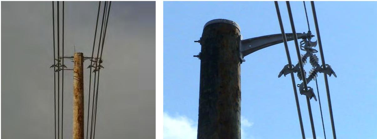
Figure 23: Covered wire with support wire
