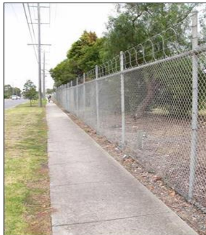
Figure 3: Pipe rail security fence to AS 1725.1 with barbed tape anti-climb feature
