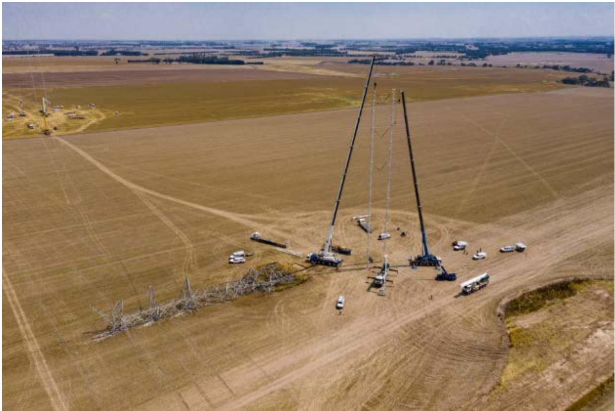
Figure 4: ERS mast structures being erected
