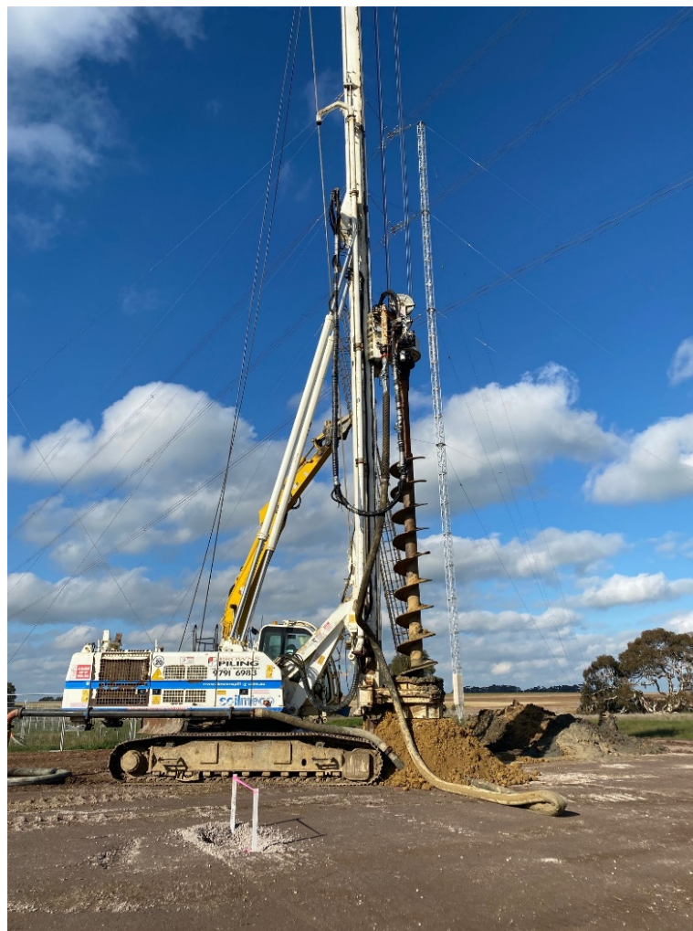
Figure 7: Foundation works for the permanent replacement towers
