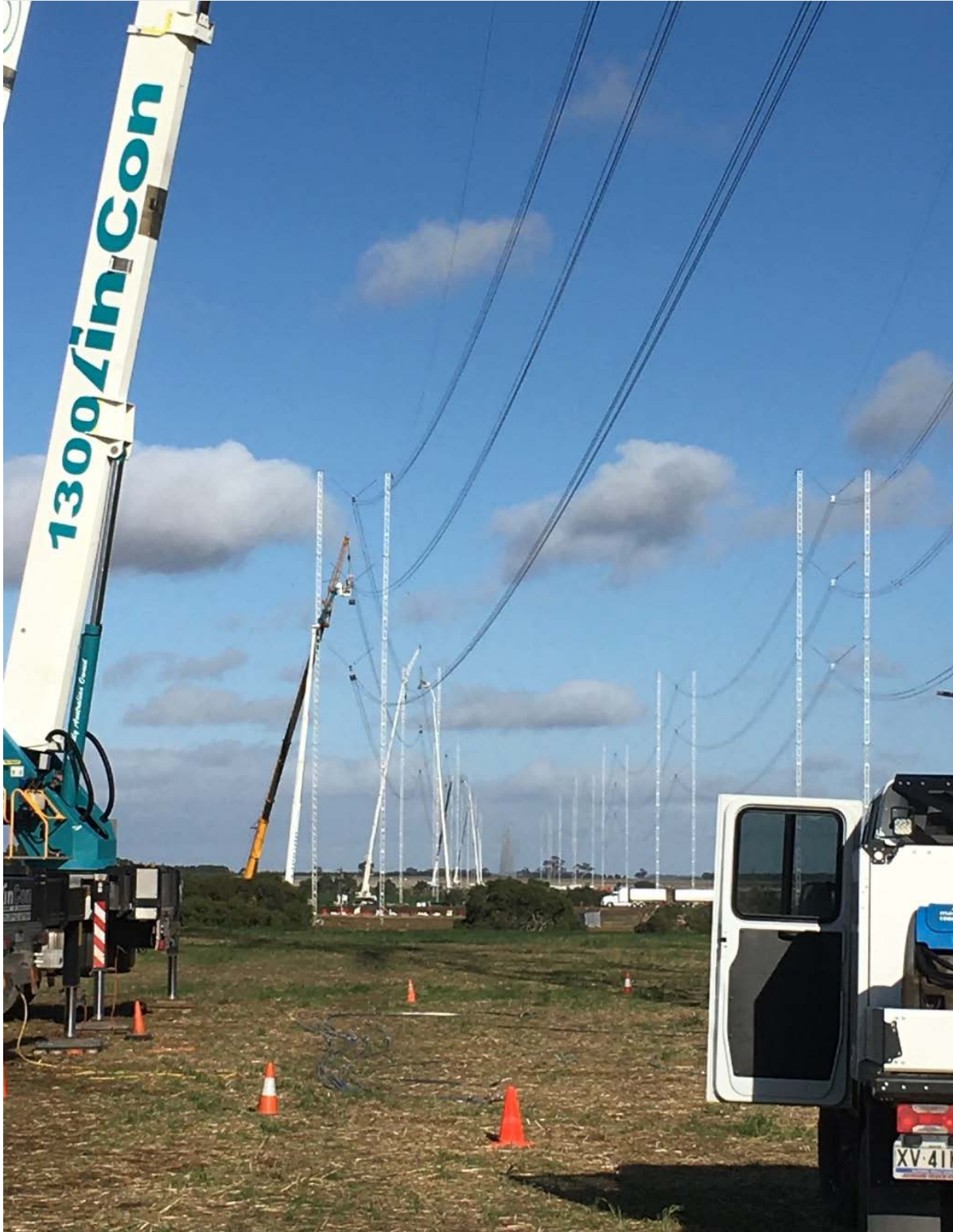
Figure 5: 2 nd bypass line being constructed
