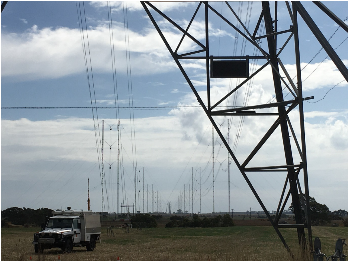
Figure 6: Completed temporary construction
