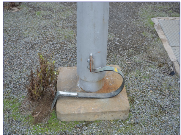
Figure 6 – Early stage of corrosion
