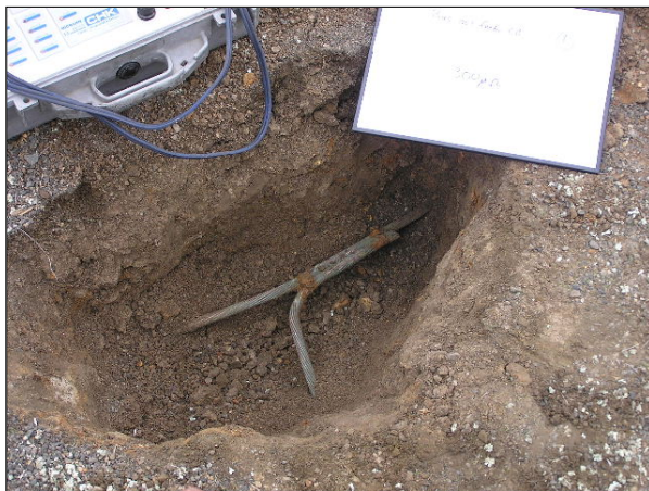
Figure 1 – Main earth grid BCC
