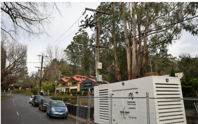
Figure 13: Mobile generation unit
