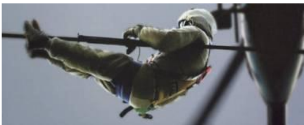
Image 3. Live Line Conductor Joint Testing
