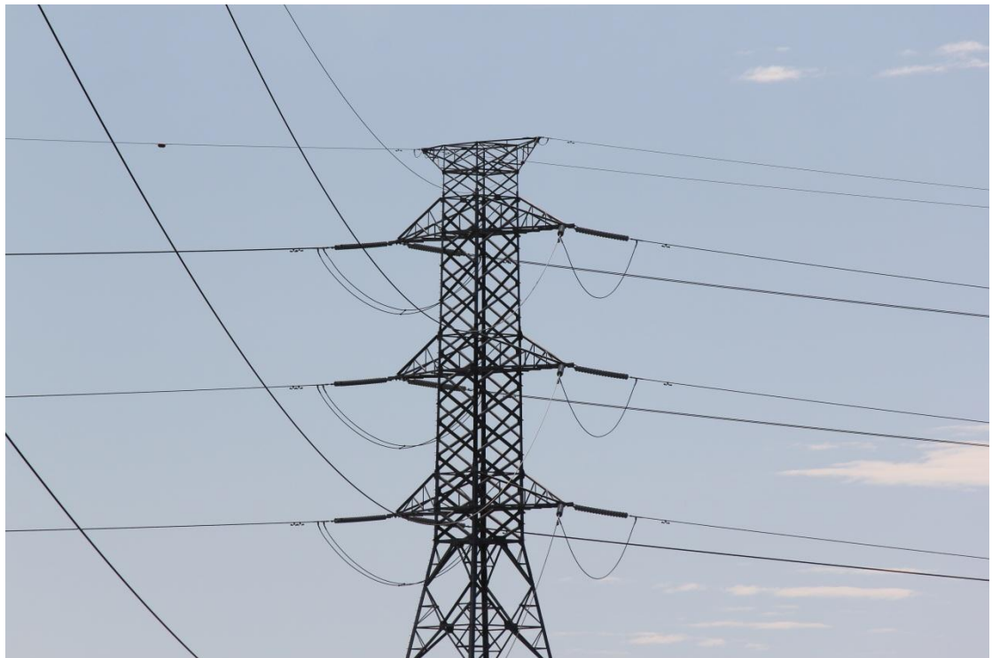
Image 5. Tension Structure
