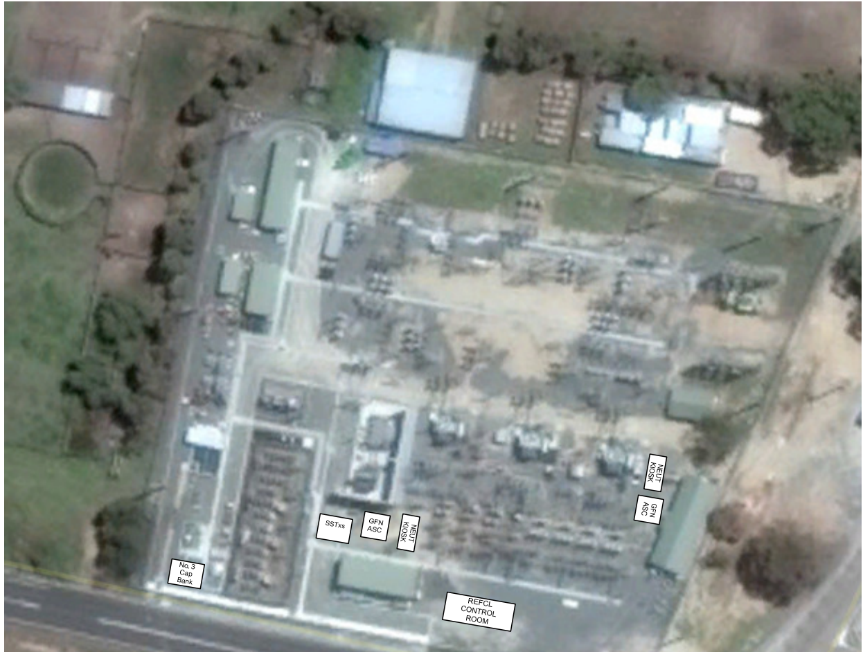
Figure 5: Aerial view of the BDL ZSS
