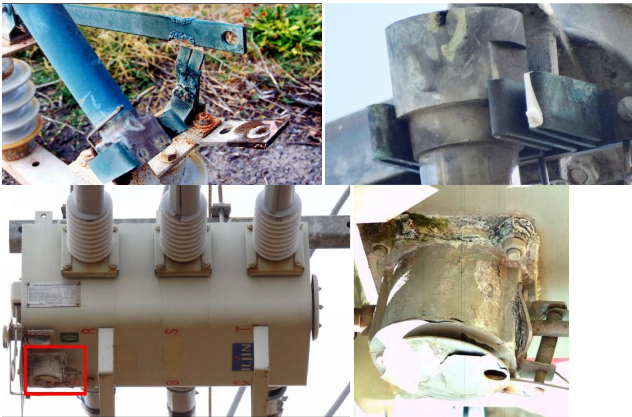
Figure 44 Typical defects of fuses and load switches
