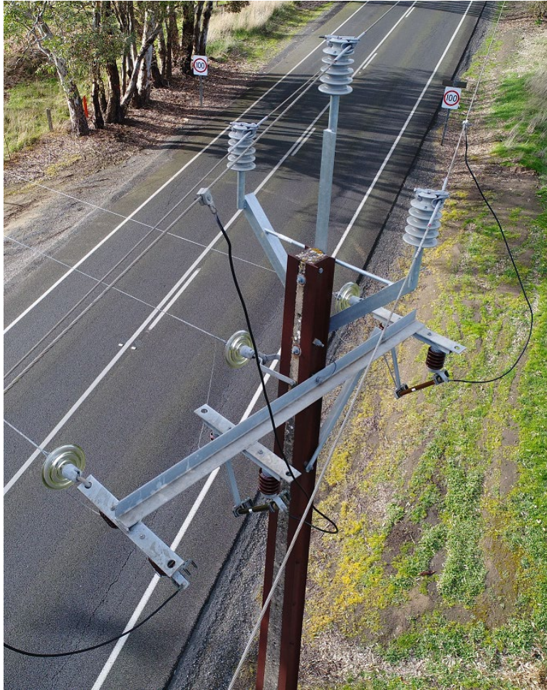
Figure 42 A typical combination of pole top structures
