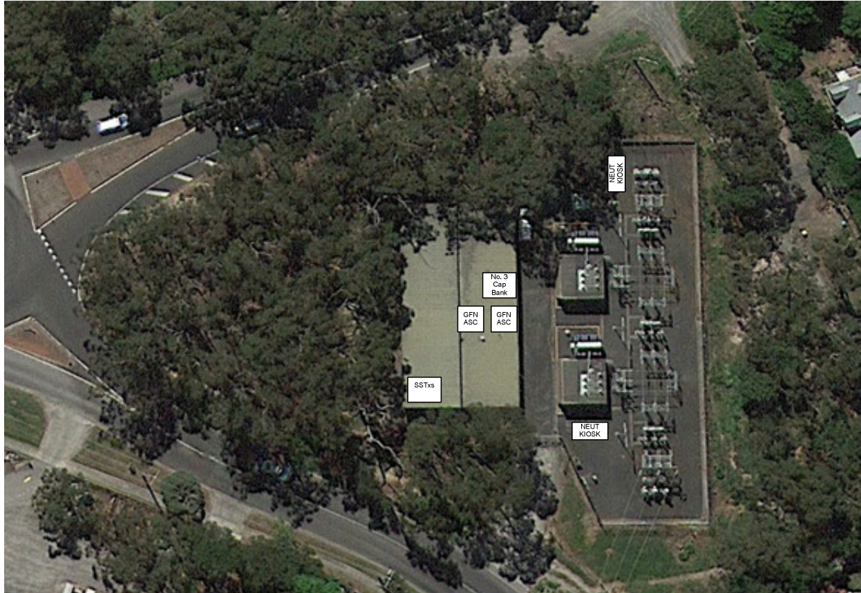
Figure 5: Aerial view of the BGE ZSS
