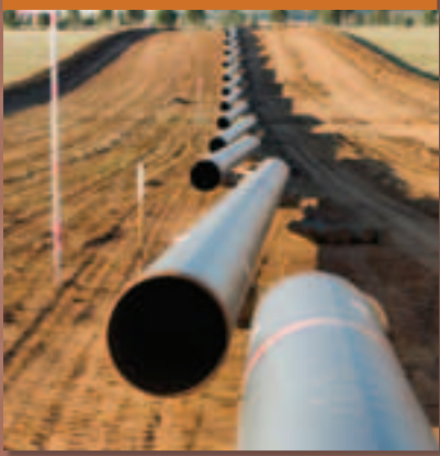
Moomba Sydney Pipeline expansion
