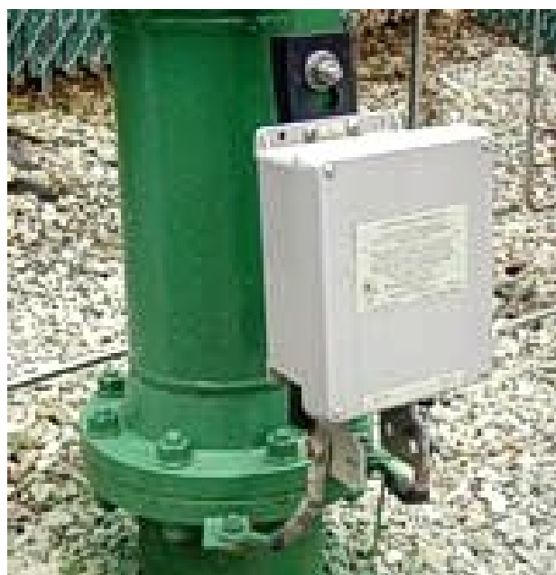
Figure 32: Voltage break over device
