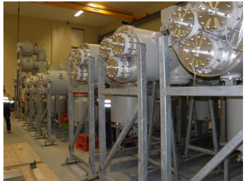
East Lake zone substation 132KV Gas Insulated Switchgear installation
