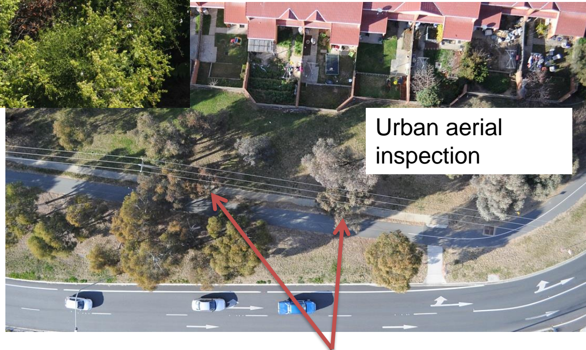
Vegetation growing into power lines
