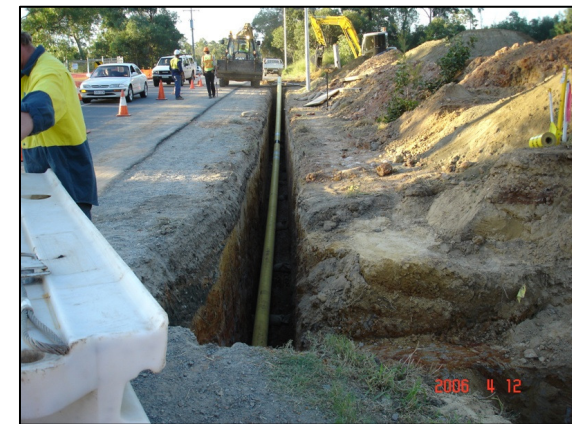
APT Allgas Network – steel main construction
