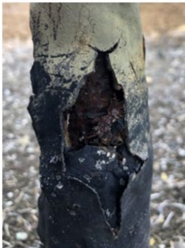
Left: Example of syphon valve corrosion where buried piping transition has failed (middle – close view) and Right: radiography to determine corrosion losses.
