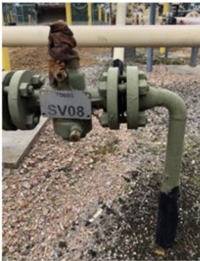
Left: Example of syphon valve corrosion where buried piping transition has failed (middle – close view) and Right: radiography to determine corrosion losses.
