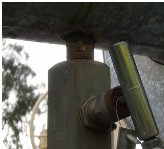
Left: Example of insulation at Dore Rd site where gaps in cladding at top instruments/nozzles allow water ingress on sweating lines. Right: Example of cladding with evidence of water ingress and corrosion at a bottom drain nozzle.
