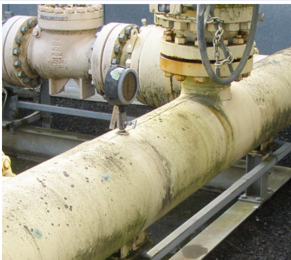
Left: Example of insulation at Dore Rd site where gaps in cladding at top instruments/nozzles allow water ingress on sweating lines. Right: Example of cladding with evidence of water ingress and corrosion at a bottom drain nozzle.
