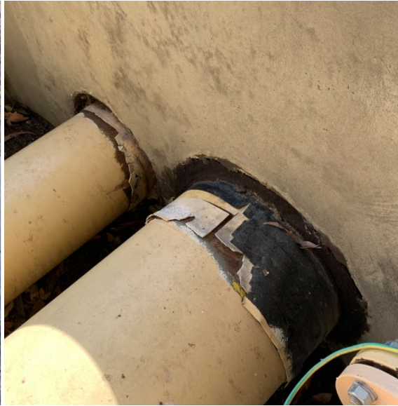
Right: Piping HDPE sleeve failing at transition in subsurface pit.
