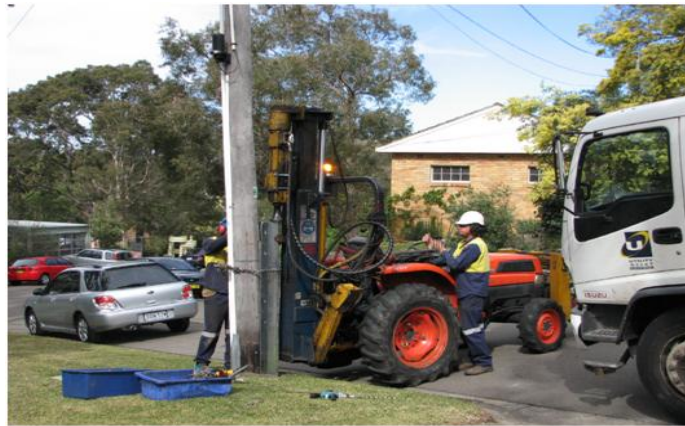
Figure 36. Pole staking - LV residential area 29
