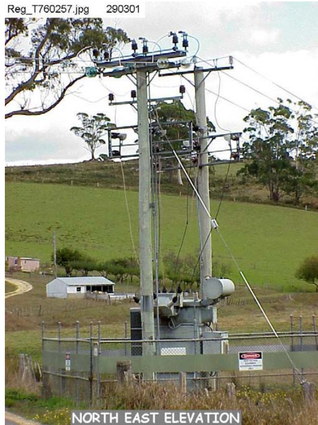
Figure 1: Typical Three Phase Regulator
