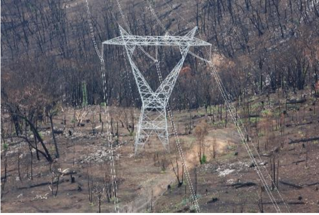
Structure 47, noting high rock content of ground, looking up number
