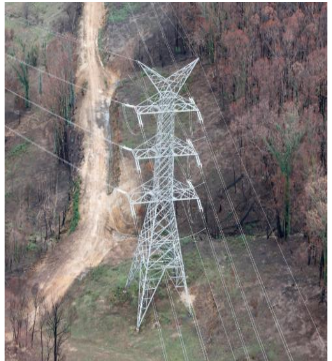
[REDACTED] Structure 7 towards 8, Pad required
