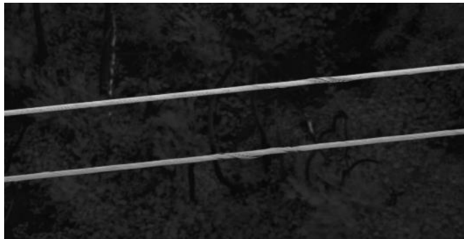
█, RHS PHz Conductor Fire Damage
