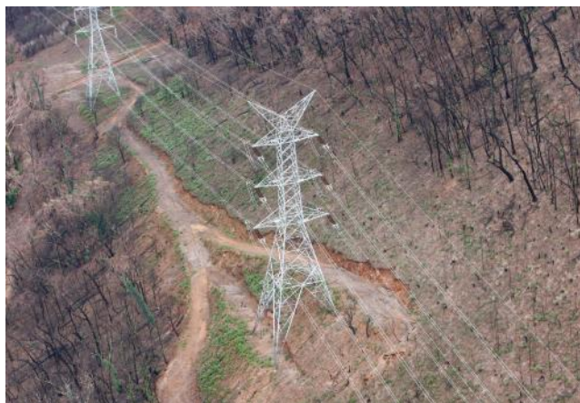
Structure 12 towards 13, Pad required
