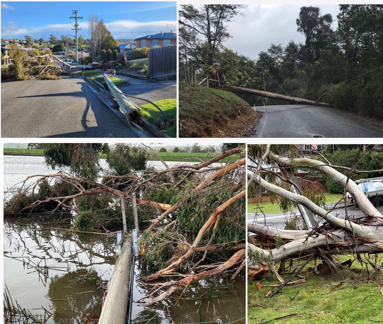
Figure 6: Examples of the extent of damage to the network
