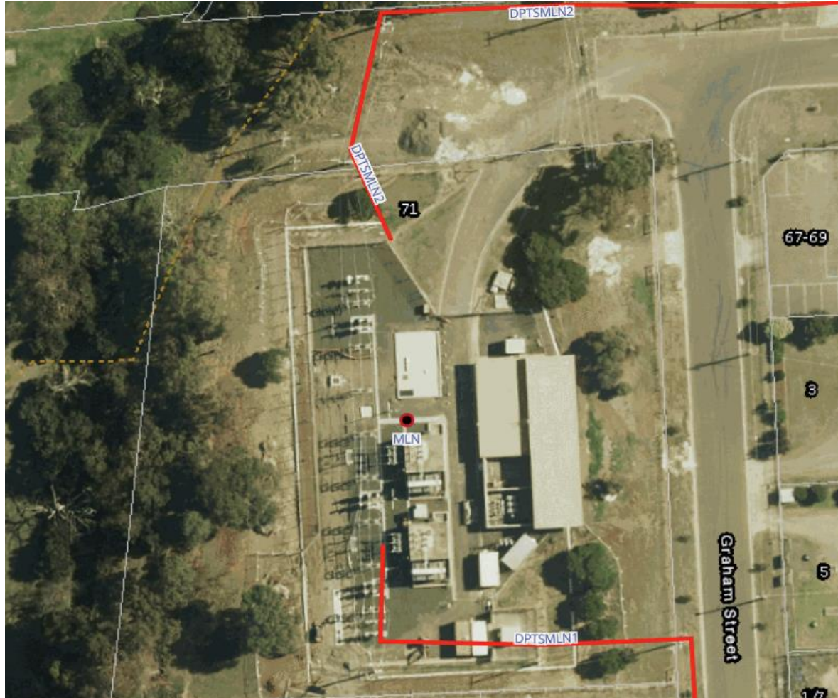
FIGURE 17 MLN ZONE SUBSTATION AERIAL VIEW
