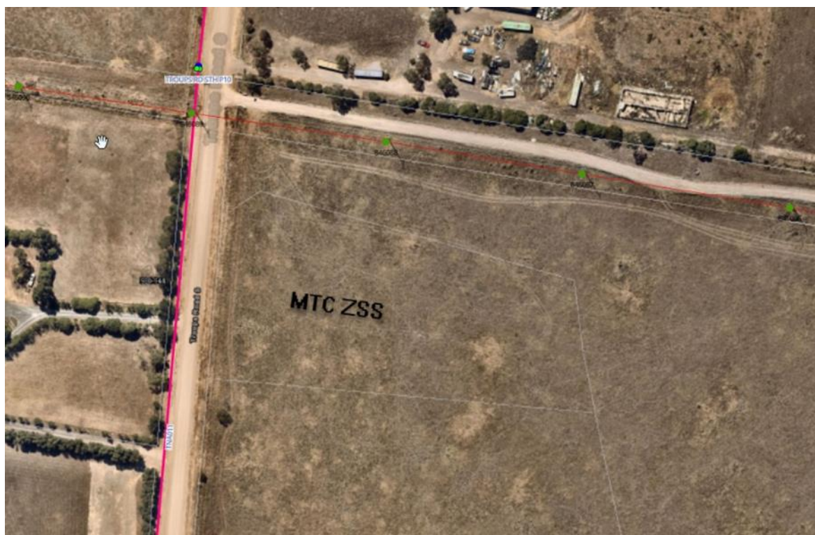
FIGURE 11 MTC ZONE SUBSTATION SITE AERIAL VIEW
