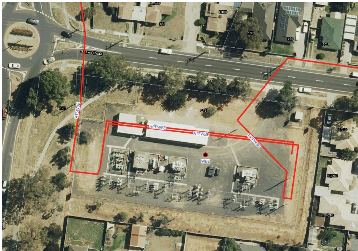
FIGURE 29 WBE ZONE SUBSTATION AERIAL VIEW
