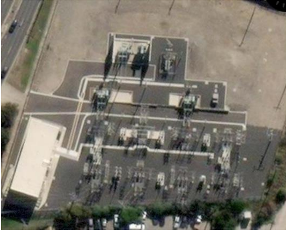
Figure 1-11 SBY Aerial View
