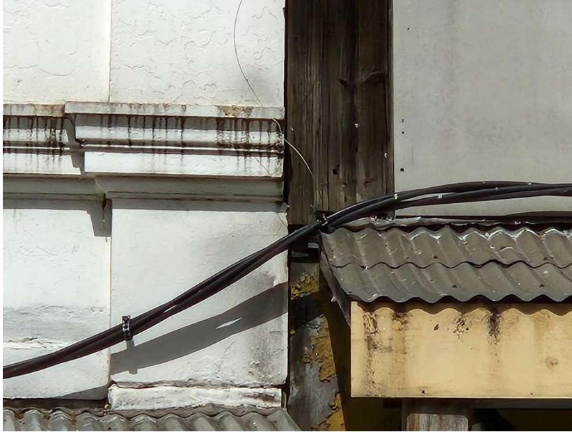
Figure 2-1: ABC Mounted On Façade
