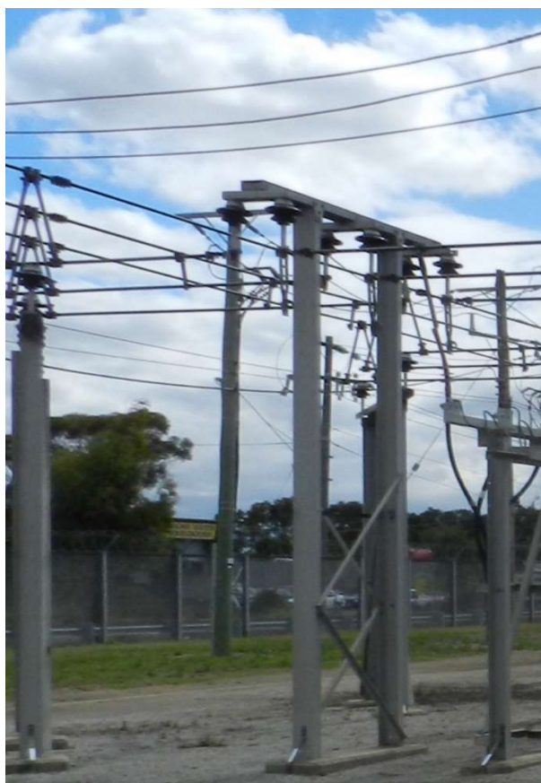
Figure 2-4: CN 22kV Transfer Bus
