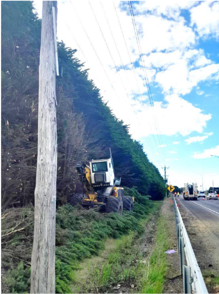
All terrain Jaraff removing a huge amount of vegetation from challenging cypress hedge spans on Drysdale zone substation
