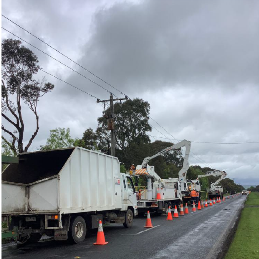
Cutting underway in September 2022 on Terang zone substation
