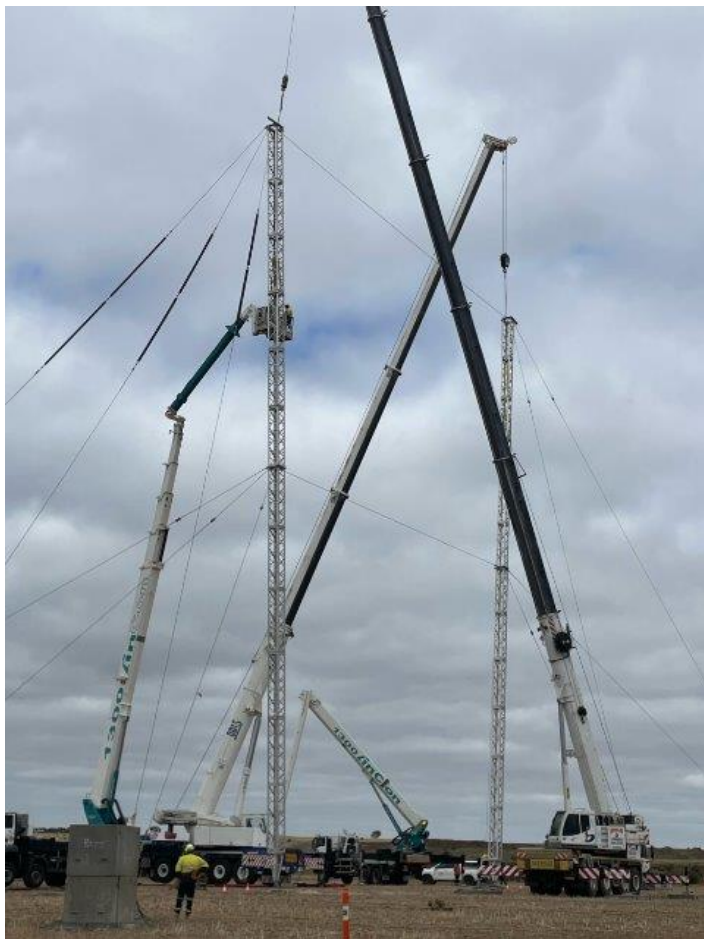
Figure 4: Emergency Restoration System being erected to temporarily restore the lines
