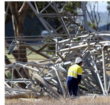
■ A worker inspects a damaged transmission tower at Anakie, Victoria, after a storm. More than 3,100 customers remain without power a week after the storms.
