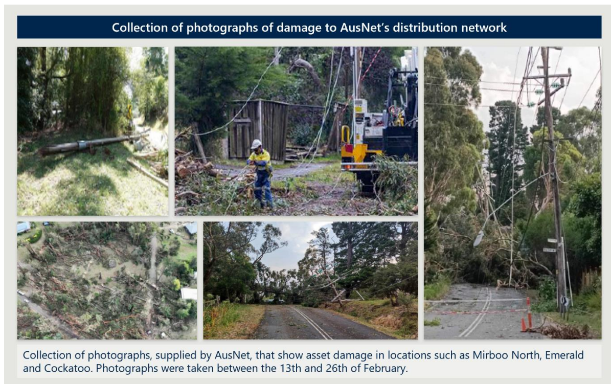
Figure 5 | Images that showcase the terrain around AusNet's distribution network and the damage caused by the February 2024 storms
