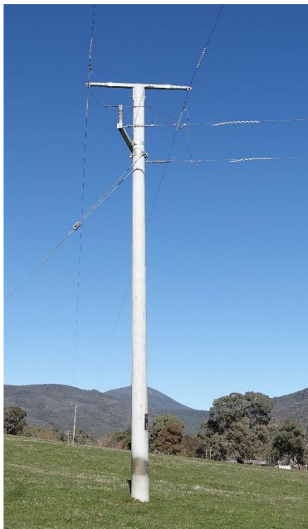
Figure 5 – Typical Glass Reinforced Concrete Pole
