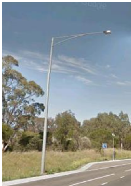
Figure 4 – Typical Galvanised Steel Pole
