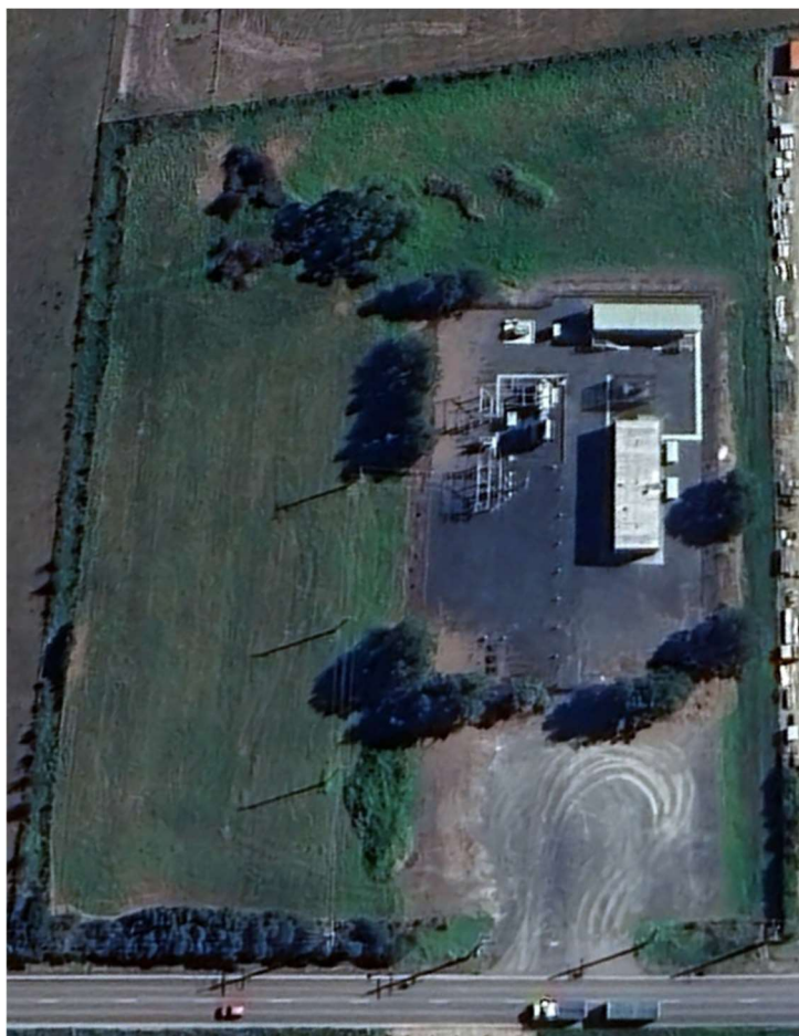
Figure 9 Lang Lang Zone Substation Site
