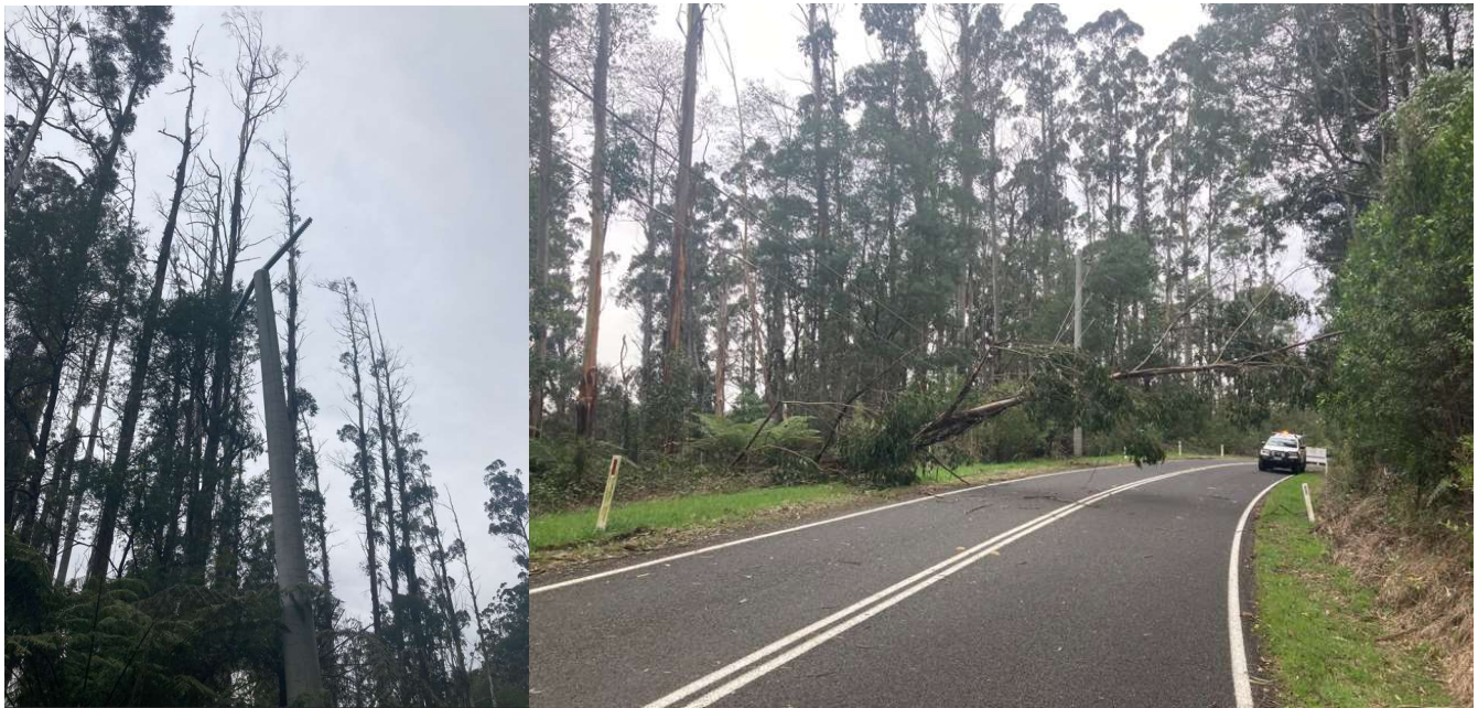
Figure 5 Photo of a hazardous tree and tree failure – Thompson Dam Rd, Baw Baw, Victoria
