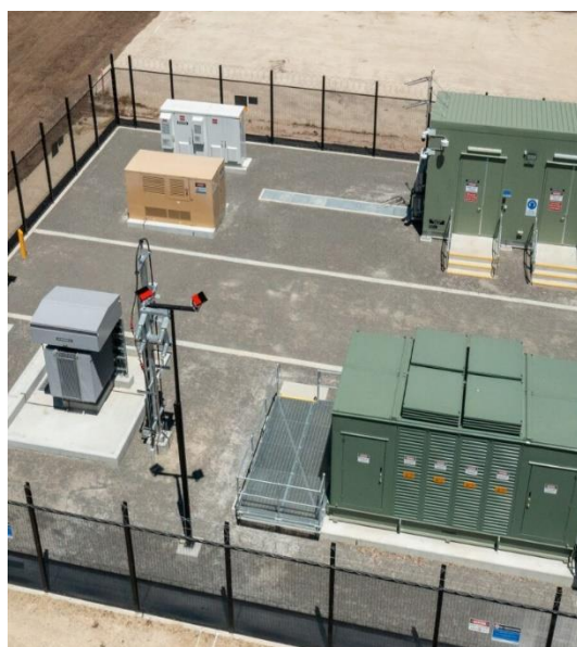
Figure 4: Aerial photo of the BNBVT Remote REFCL site.
