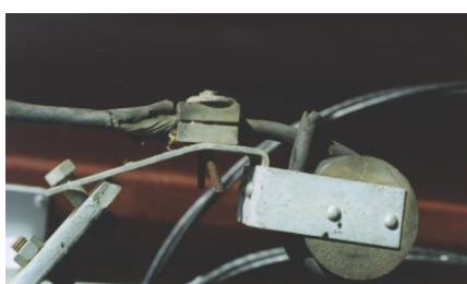
Figure 3 - Neutral Screened Service and Roller Clamp
