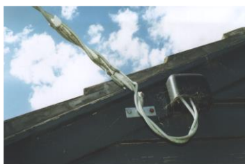
Figure 2 - Grey PVC Service and 'Dog-bone' Termination Fitting
