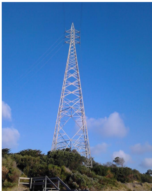
Figure 3: San Remo Tower
