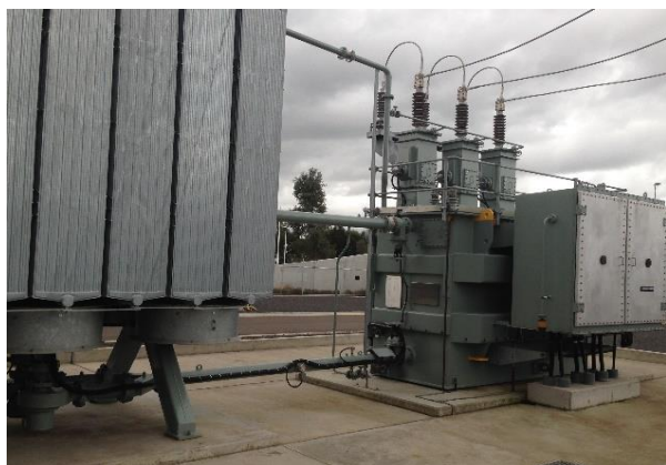
Figure 8 - Concreted bunded area at Bayswater zone substation (BWR)
