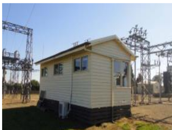
Figure 6 - Wood board clad control
