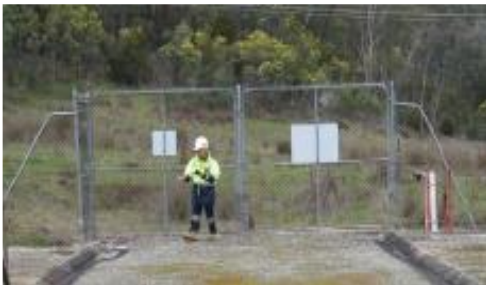
Figure 8a - Security fence & gate at Mt. Beauty zone substation (MBY), before augmentation
