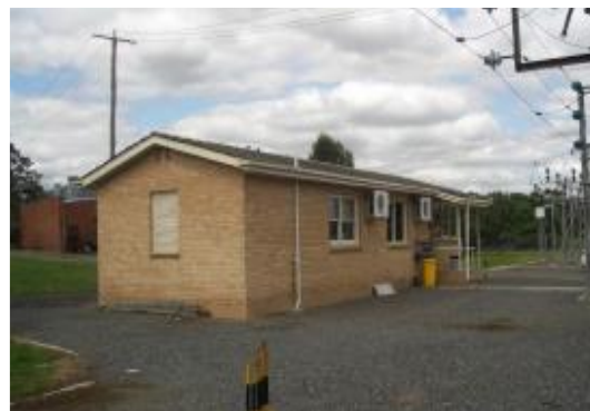
Figure 4- Brick control building at Croydon zone substation (CYN)
