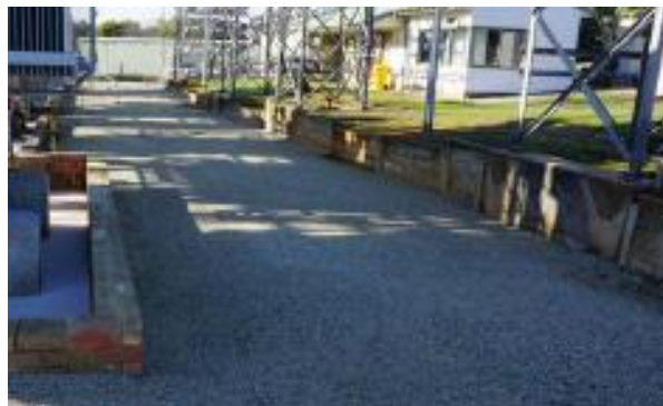
Figure 10 - Access Road surface located at Warragul zone substation (WGL)
