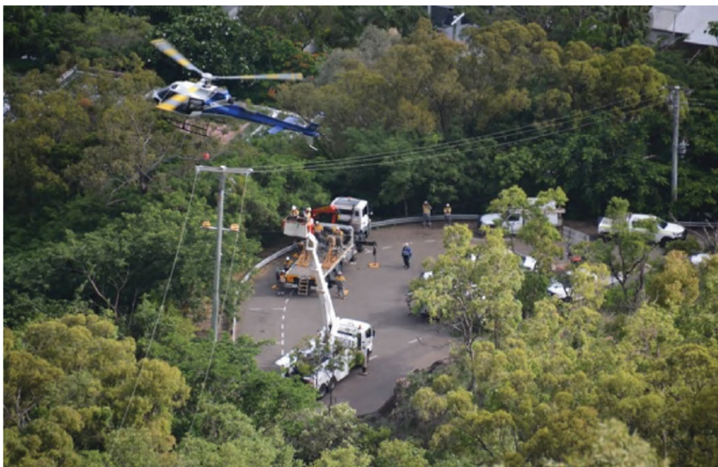
Figure 4: Re-stringing of fallen powerlines on Castle Hill
