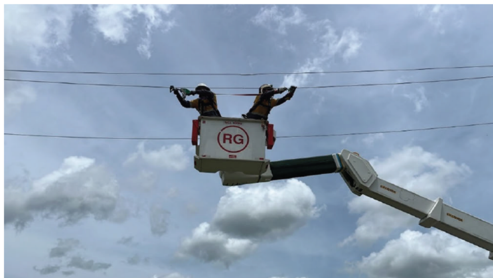
Figure 5: Ergon Energy crews completing post-cyclone repairs
