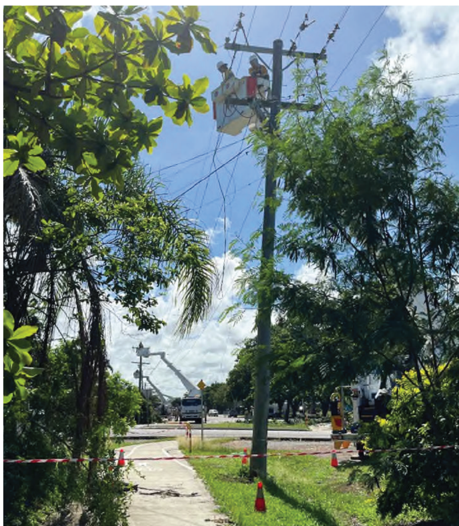
Figure 6: Ergon Energy crews and trucks completing street long repairs
