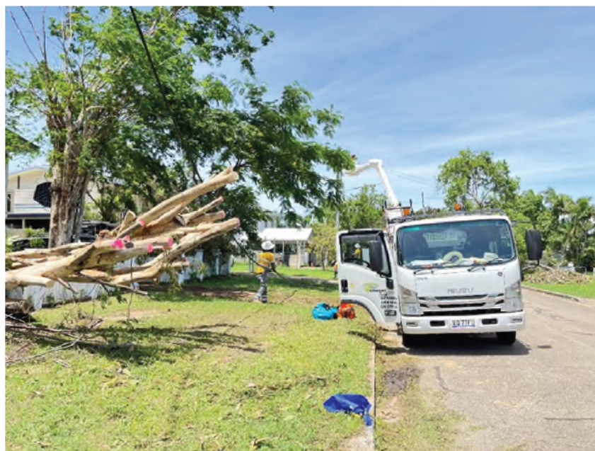
Figure 10: Crews working to repair damage to the network in Townsville
