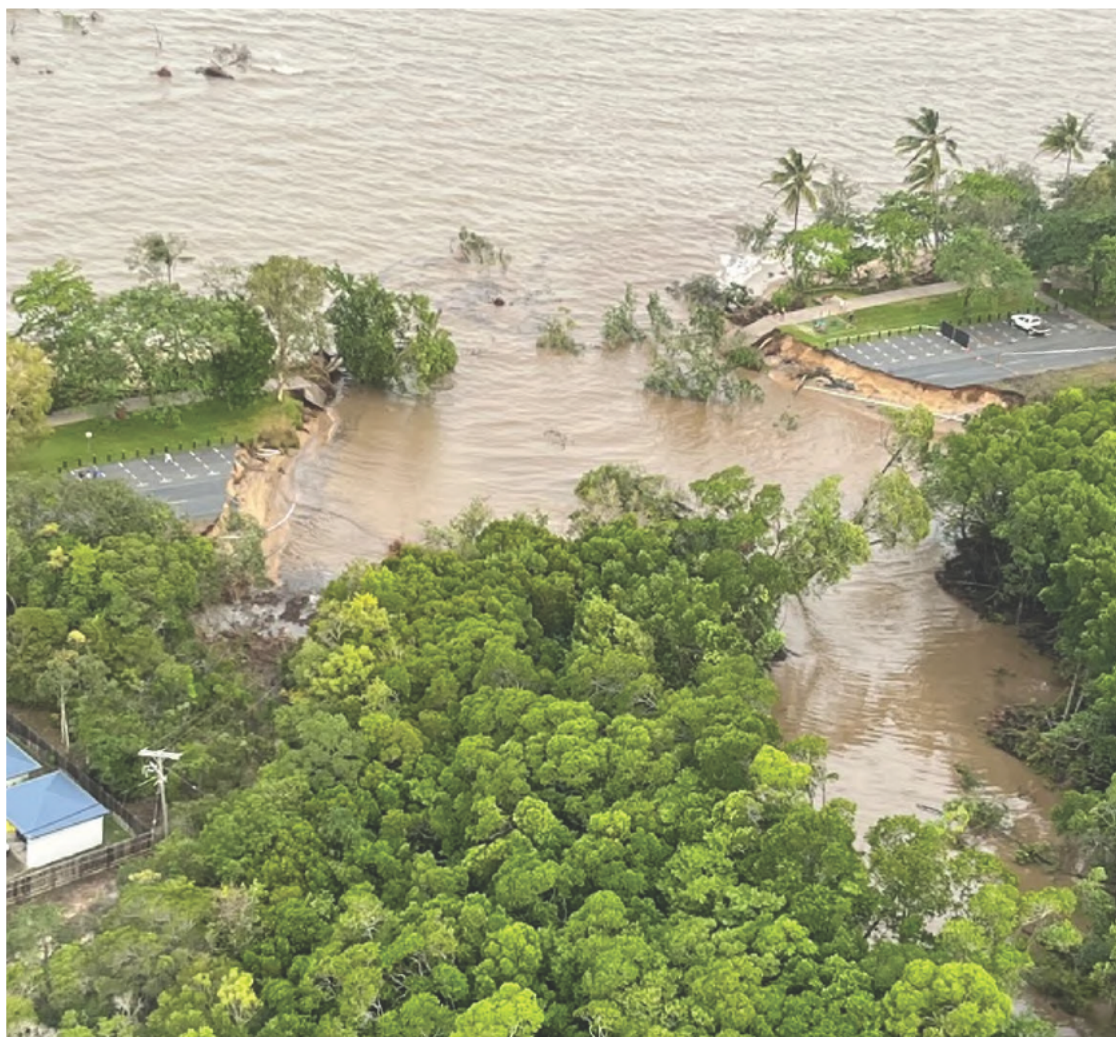
Figure 6: Flooding and Infrastructure damage in Holloways Beach
