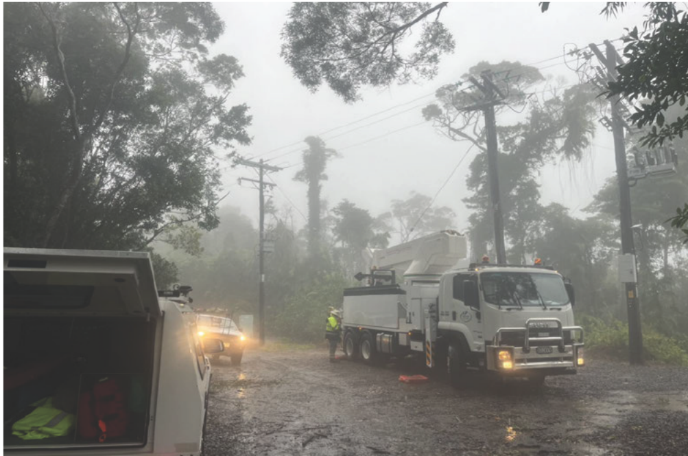
Figure 4: Ergon Energy crews completing post-cyclone repairs in difficult conditions
