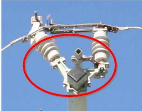
Figure 9 - ABB "U" Series Powder coated aluminium bracket
