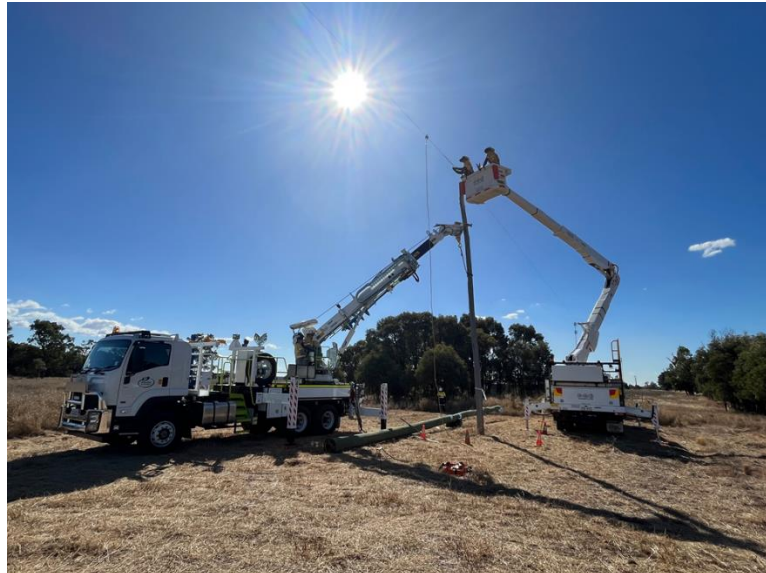
Figure 1: Example crane borer in operation
