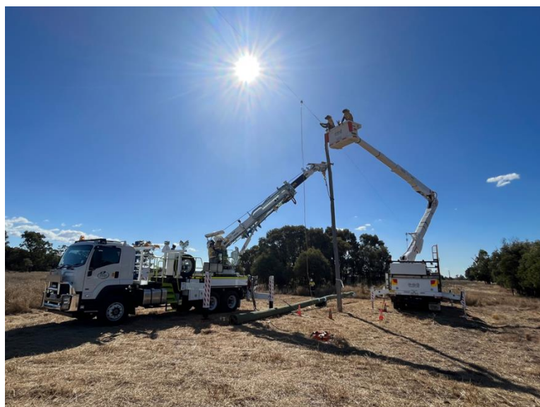
Figure 1: Example crane borer in operation
