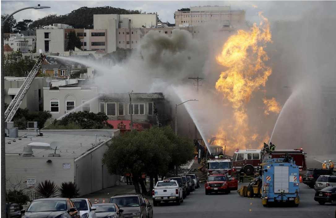
Figure 2 Wednesday, Feb. 6, 2019. A 4-inch plastic gas pipe explosion in San Francisco.
