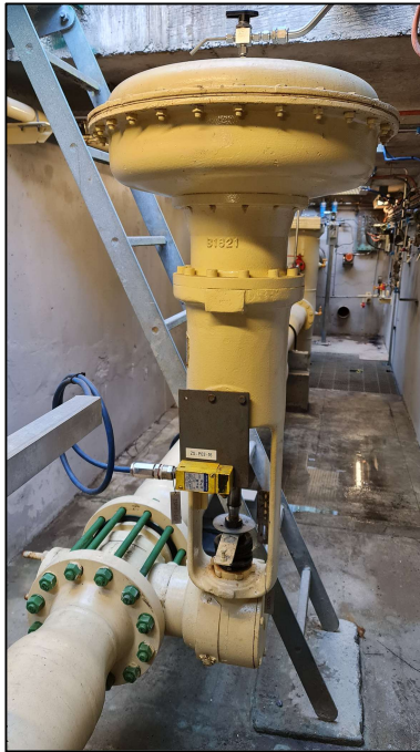
Figure 8 : Control Valve Regulator
