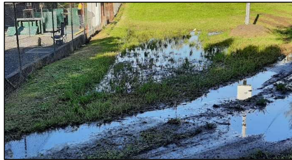
Figure 5 : Site vehicle path to exit site after rain event
