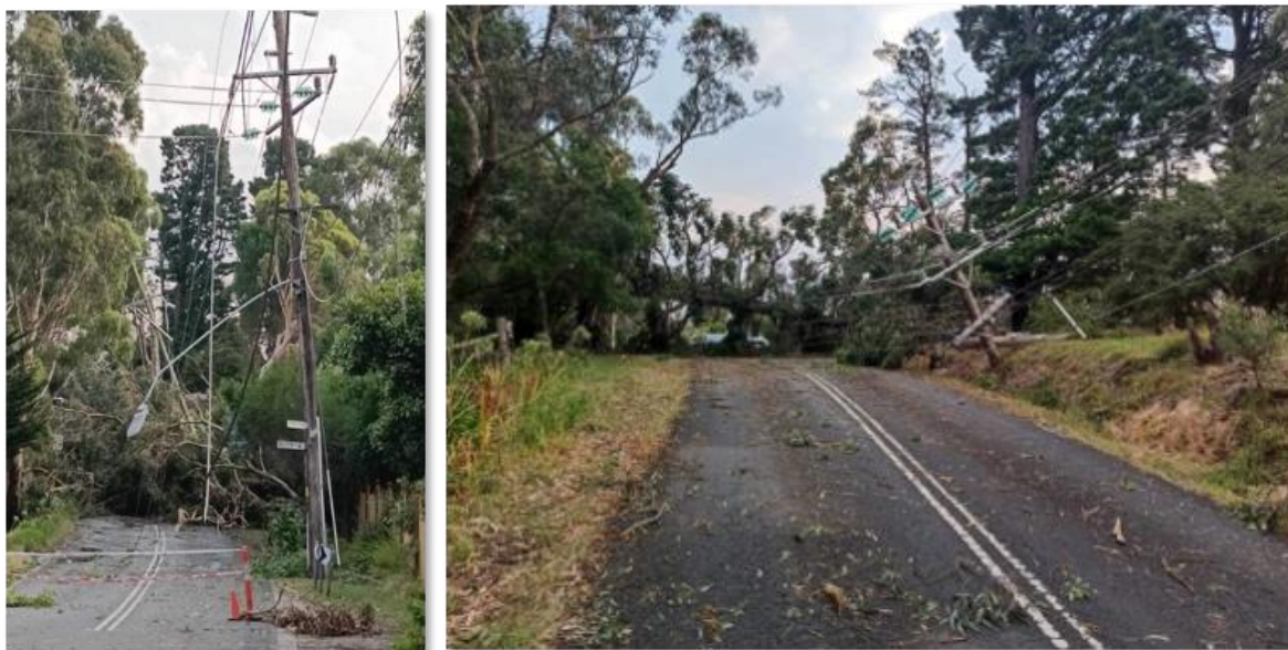
Figure 2: Examples of damage to our networks as a result of the February storm
