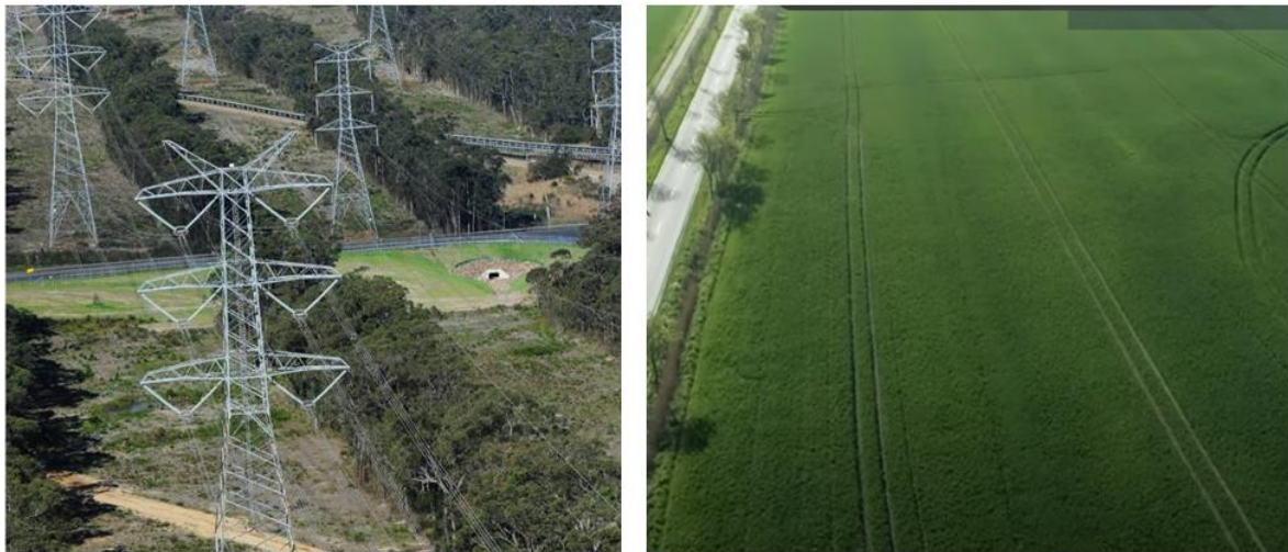
Figure 3: Landscape character and land use impacts of overhead lines and underground cables
