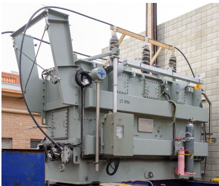
Substation transformer
