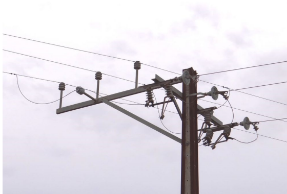
Pole top structure
