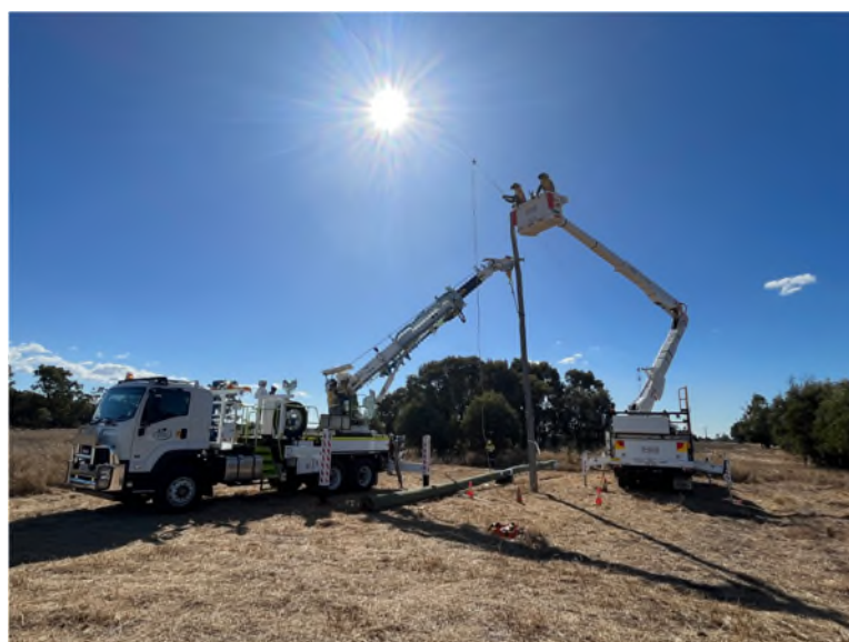
Figure 1: Example crane borer in operation
