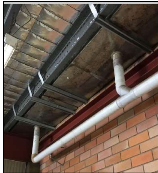
Building B – Internal guttering & ducting
